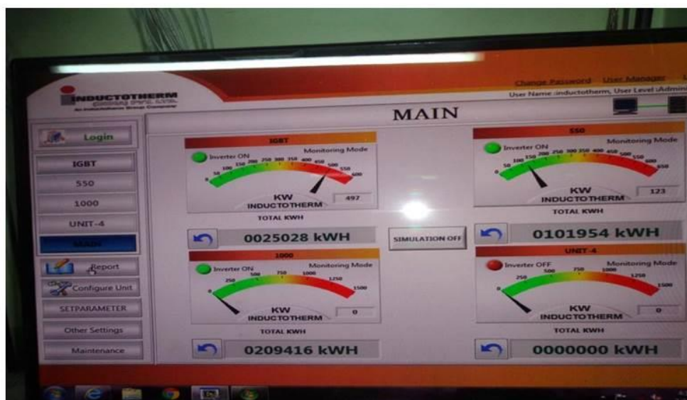
Installation of induction furnace energy monitoring system
